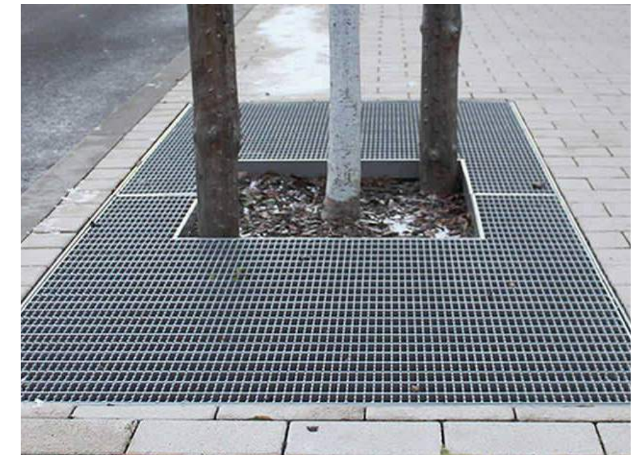
Open bar grating at tree wells.
