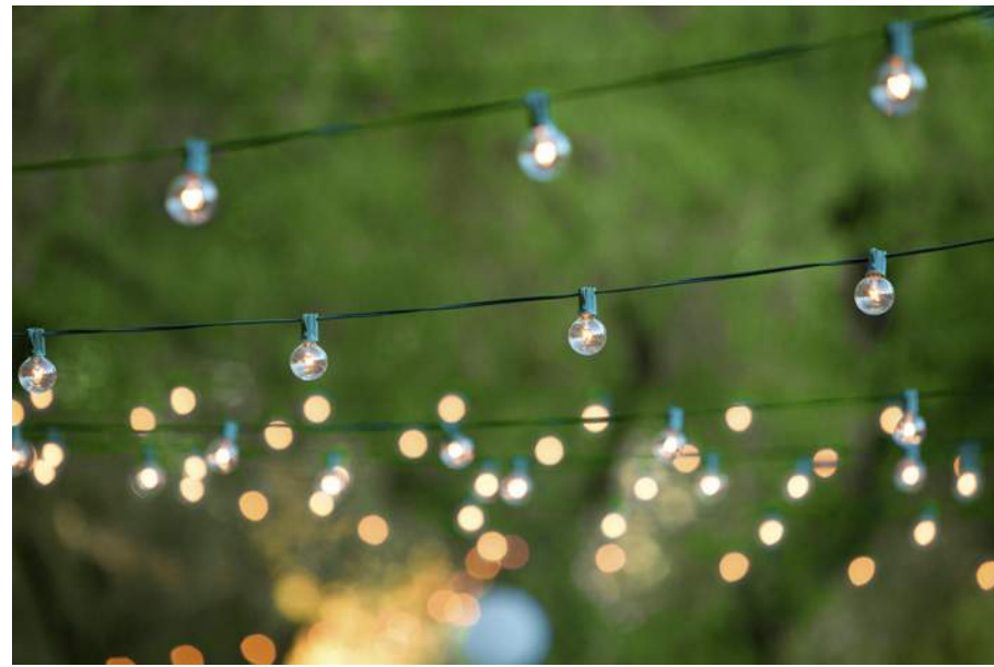
Catenary lights at the residential outdoor amenity area.
