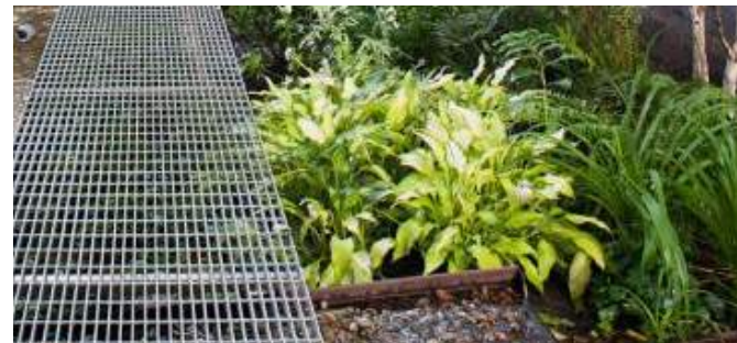
Open bar grating at tree wells.
