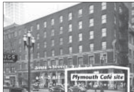
The St. Charles is already undergoing extensive renovations, including the addition of Plymouth Café.
